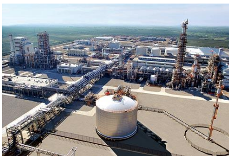
Fertilizer manufacturing plant (Turkmenistan)
