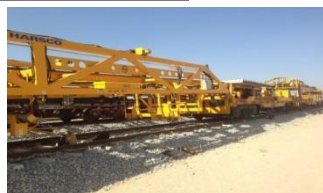
Laying of head hardened rails
