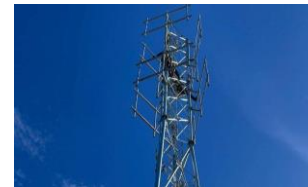
Telecommunications Tower Business in the Philippines
