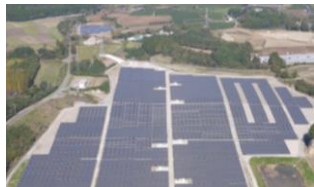
Solar Power Plant in Nishikimachi, Kuma-gun, Kumamoto
