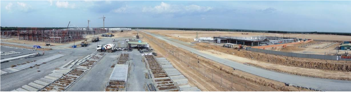
Construction works in the Long Duc Industrial Park
