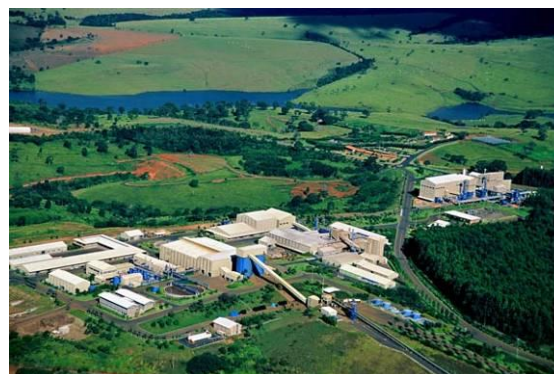
Niobium refining plant in Brazil
