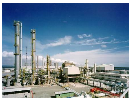
-Methanol manufacturing plant in Indonesia
