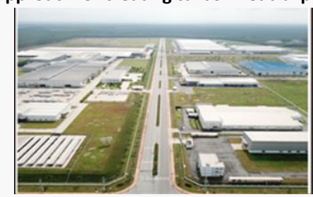
Image of Industrial Park
