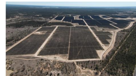
Completed Edenvale Solar Park in Sep. 2023
