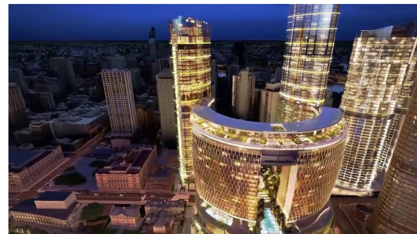
Energy Saving Service Business (Australia)
